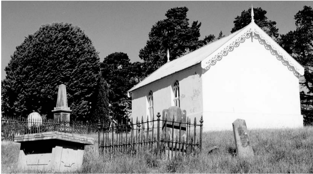
Kirklands Church north west of Campbelltown in Tasmania, built in 1836. (photo: Cameron Archer)
