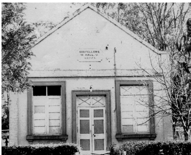
The Paterson Oddfellows Hall prior to additions (photo: Geoff Keppie)
