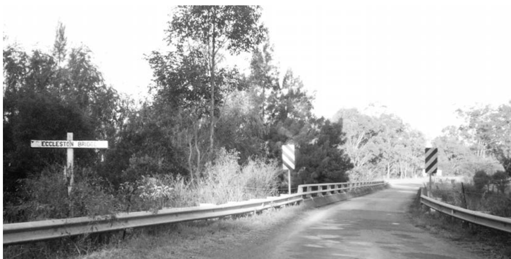
Eccleston Bridge, Allyn River. Ravenscroft Chapel was on the northern side of this river crossing before it was swept away in the 1875 flood (photo: Cameron Archer)
