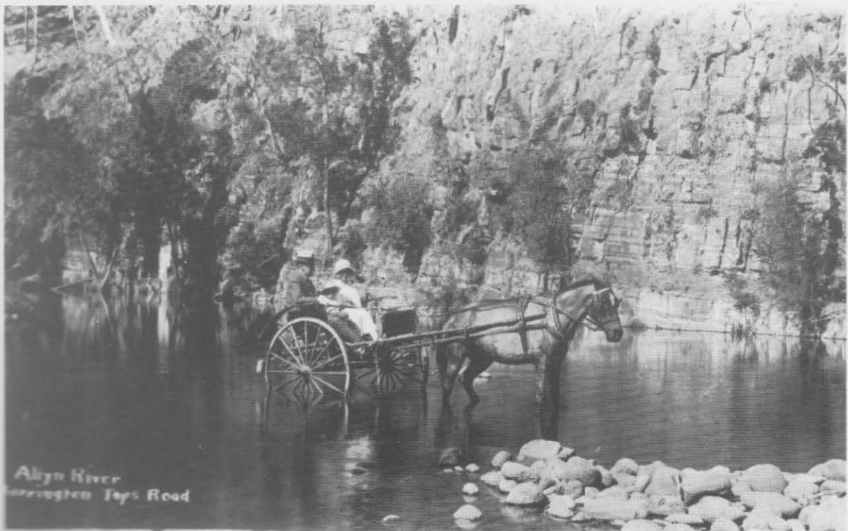
Allyn River Crossing – Barrington Tops Road
