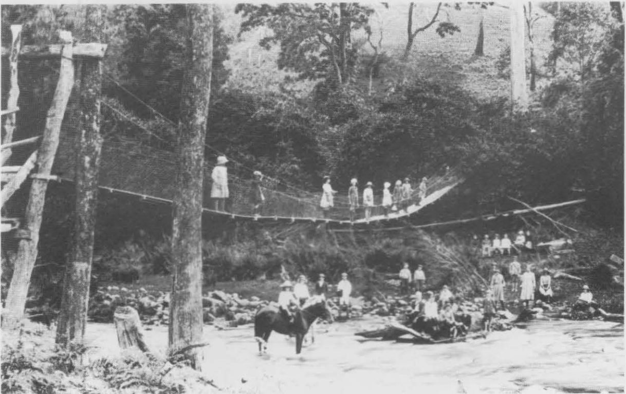
Suspension Bridge – Allyn River – Eccleston
